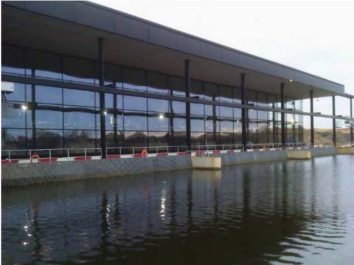
St Germans Pumping Station Source: Middle Level Commissioners
